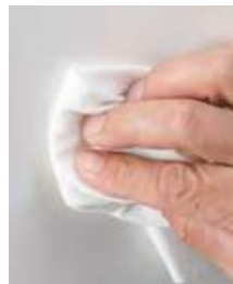
6. REMOVE ADHESIVE RESIDUE
